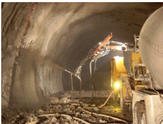
Fig.9 Shotcrete construction using cement mineral type accelerator
