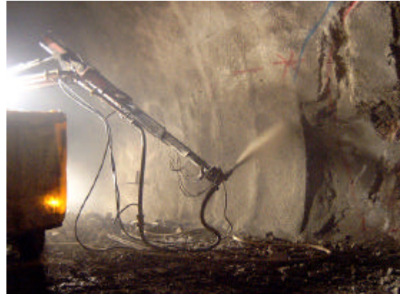
Fig.9 Shotcrete construction using cement mineral type accelerator
